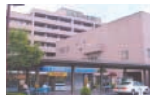
LAWSON outlet at Kanto Chuo Hospital
