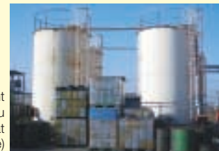
Eco-Town Recycling Plant in Kitakyushu (Kyushu Yamaguchi Oil and Fat Industry Cooperative)
