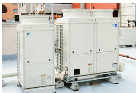
Energy-Saver Pack outdoor unit for new stores
