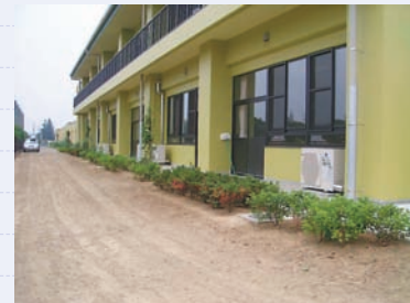
Shrubby additions around buildings constructed to house an influx of students at the Ota School for the Disabled in the city of Ota, Gunma Prefecture
