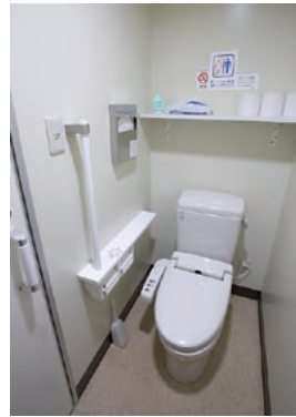
Western-style toilets with safety handrails
