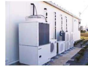
Outdoor units of CO 2 coolant
