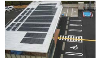
Solar power system on the roof of our store in front of Panasonic head office
