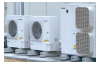
Approximately 3,400 stores have introduced CO 2 refrigeration systems (as of end February 2019).
